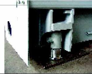
Rocker Pin Construction: Proven Design, Simple to Install, and Maintain
